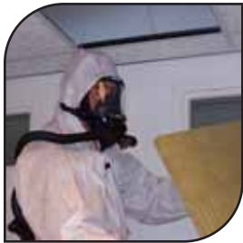
Asbestos Stripping
